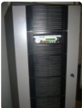
Lot: 601 PowerWave 5000/T UPS cabinet: 7.5 - 40kVA, 3-phase (excl battery)
