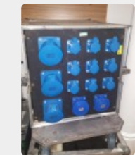
Lot: 262 14-Way Power Distribution: 16A & 63A outputs built into wheeled flight case
